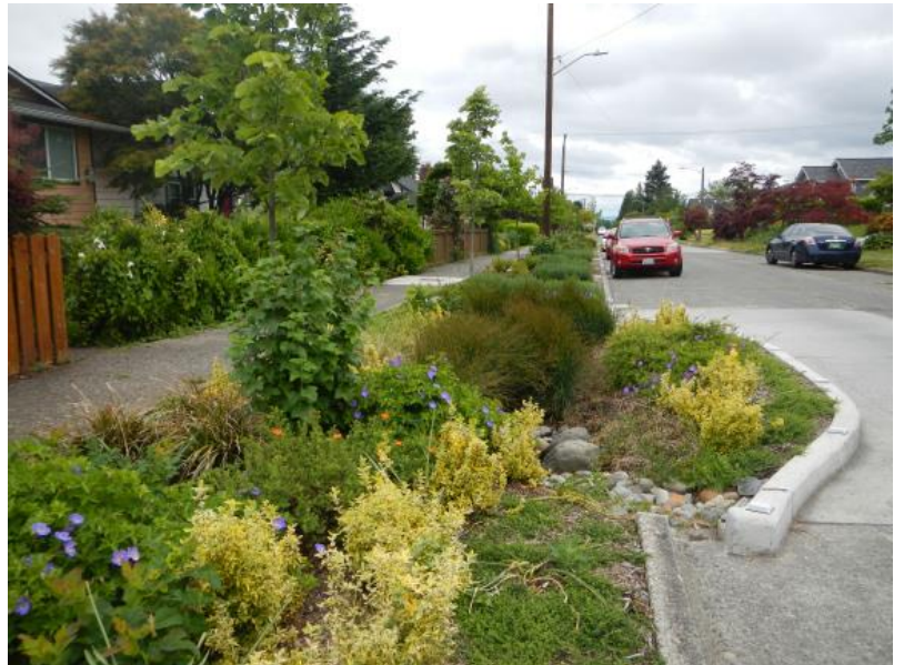
Example of a roadside rain garden
