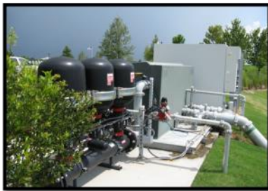
Stormwater Harvesting and Recycling (Sarasota, Florida)
